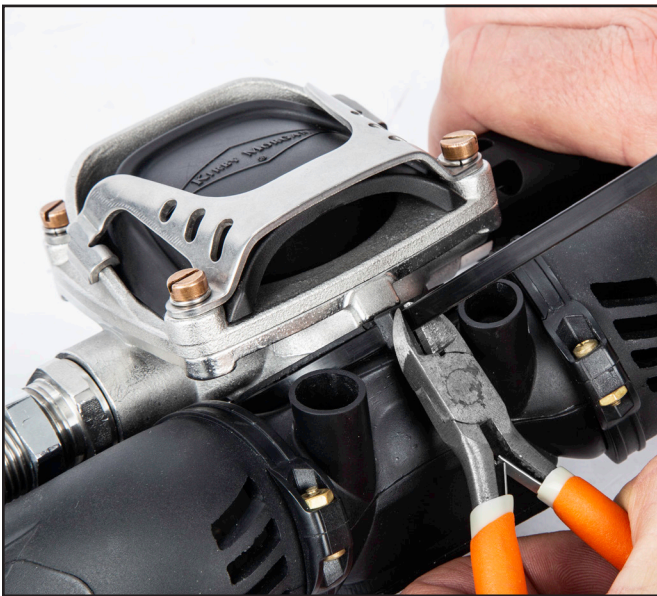
Remove excess tie wrap.
