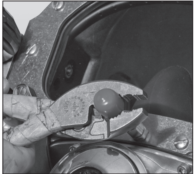
Protect the nose block device knob with a plastic cap or rag when you remove it.
