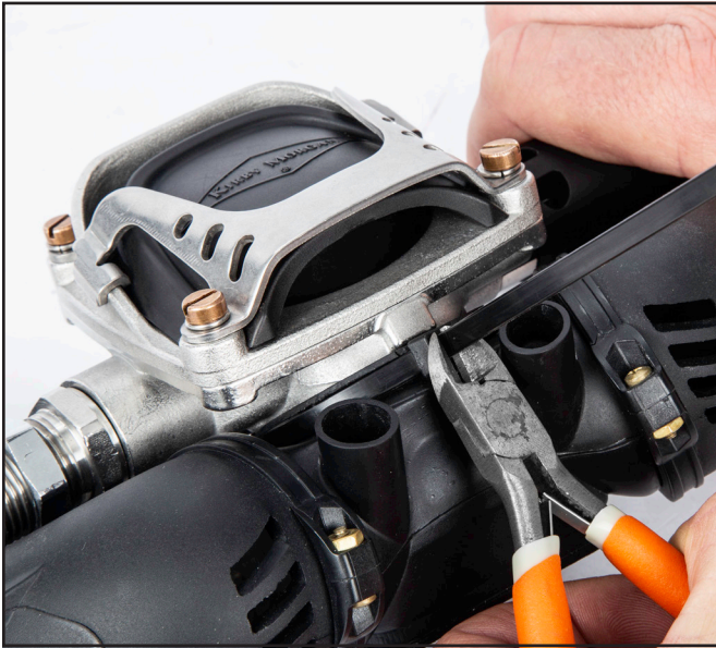
Remove excess tie wrap.
